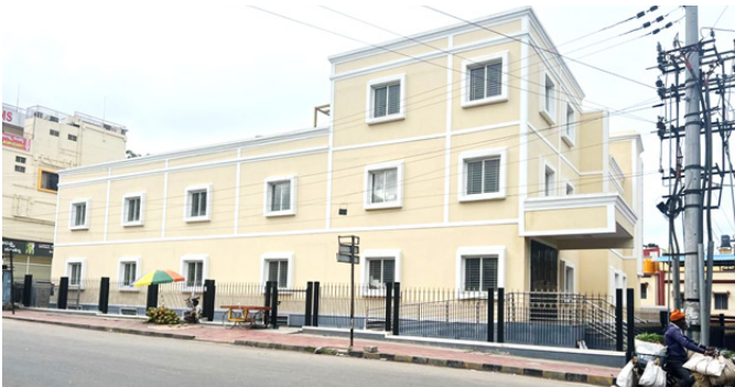
The building which was supposed to become Regional Passport Kendra in Mysuru.
