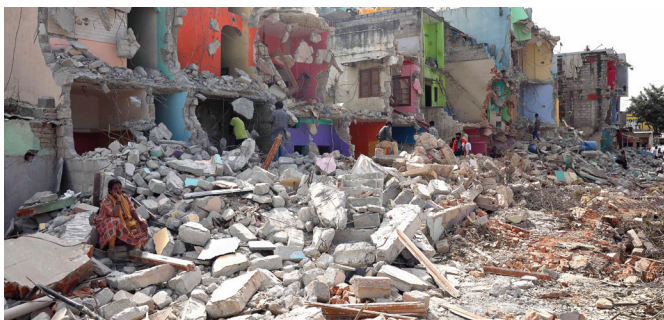
Residents were seen rebuilding their lives on Monday after authorities demolished their homes. ▸ CH PHOTO
