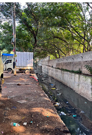
An unbarricaded, open rajakaluve canal on Jasma Bhavan Road—running right beside the main road. Right next to it is the KPCC Office where official vehicles regularly park—poses a fatal hazard for pedestrians. Lacking retaining walls or proper street lighting, the gaping drop threatens to sweep anyone into the channel in the dark, prompting urgent demands for safety barriers.
