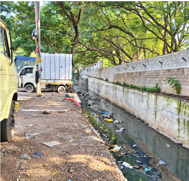
An unbarricaded, open rajakaluve canal on Jasma Bhavan Road—running right beside the main road. Right next to it is the KPCC Office where official vehicles regularly park—poses a fatal hazard for pedestrians. Lacking retaining walls or proper street lighting, the gaping drop threatens to sweep anyone into the channel in the dark, prompting urgent demands for safety barriers.
