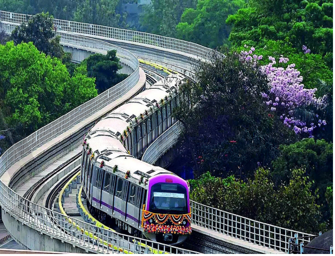
Namma Metro’s 44.65-km Orange Line takes a key step forward with BMRC seeking global consultants for project implementation.
