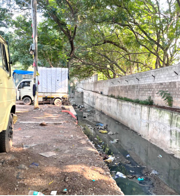
An unbarricaded, open rajakaluve canal on Jasma Bhavan Road—running right beside the main road. Right next to it is the KPCC Office where official vehicles regularly park—poses a fatal hazard for pedestrians. Lacking retaining walls or proper street lighting, the gaping drop threatens to sweep anyone into the channel in the dark, prompting urgent demands for safety barriers.
