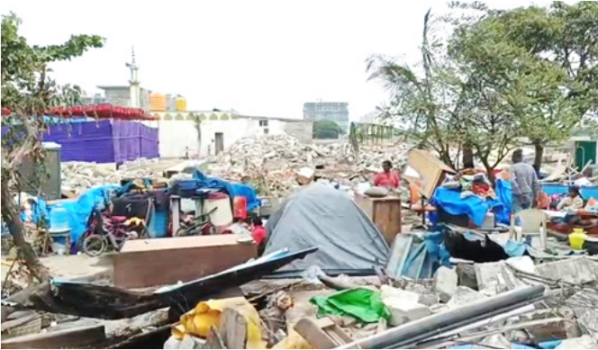
Our houses were demolished without any proper notice, under heavy police protection. We were helpless when more
