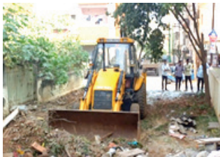
the illegal structures erected across the public road were demolished, thereby restoring unhindered access for public use. Approximately 6,000 square feet of land worth around Rs 10 crore has been reclaimed by the City Corporation. Further legal action will be initiated against the individuals responsible for the encroachment as per applicable provisions. The operation was carried out under the supervision of the EE and AE of concerned division.
