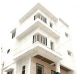
connection is being hampered. Although exemptions were given for buildings with an area of 30x40, residents are now stuck in a bind. Electrical contractors say this is a problem in thousands of buildings. The government has given permission for only three floors in total. Even if a small bathroom or store room is built beyond three floors, permission is not given. Contractors are insisting that such buildings be considered. Overall, the government has exempted OC for 30x40 buildings. In addition, the rule of G plus two or stilt plus three floors should be relaxed a little for already constructed buildings. People and contractors are complaining that this will cause a lot of problems.
