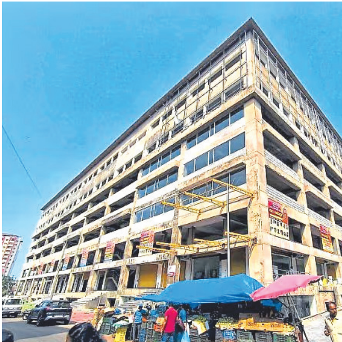
six-storey structure with a total area of five lakh sq. ft.
