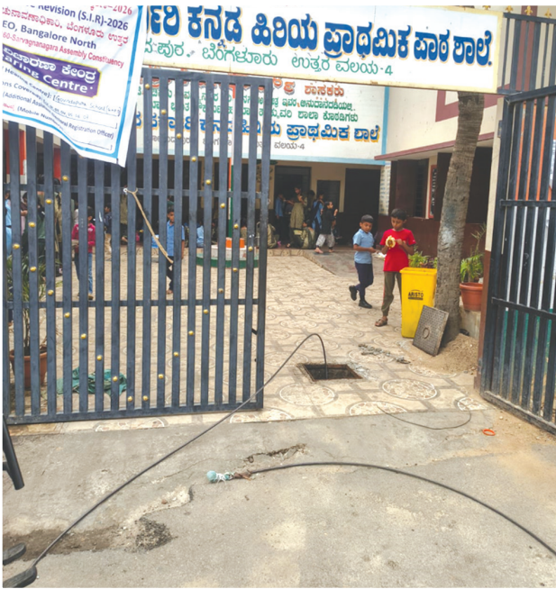
At Govindapura Government School, also serving as an SIR hearing center, an open pit on campus threatens playing children and nearby lunch services.
