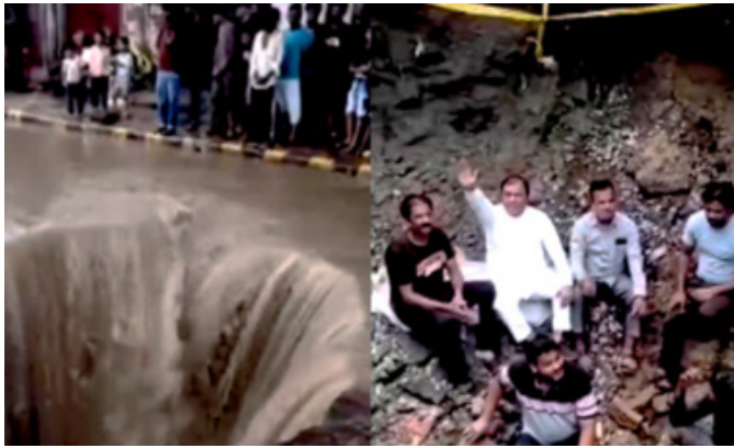
SP MLA Hasan Roomi entered an 18-foot-deep road pit in Kanpur to protest poor road conditions after heavy rain caused a section of VIP Road to collapse.
