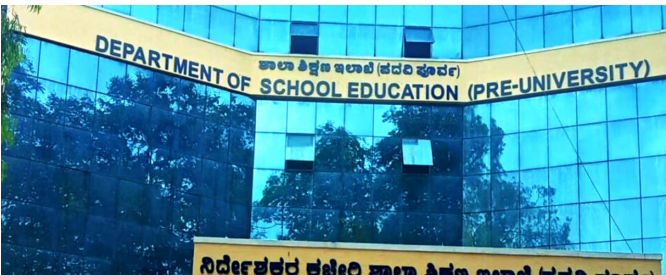
The Department of School Education (Pre-University) building.
