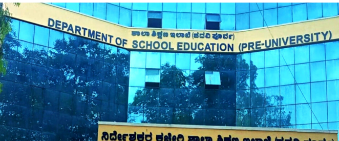
The Department of School Education (Pre-University) building.
